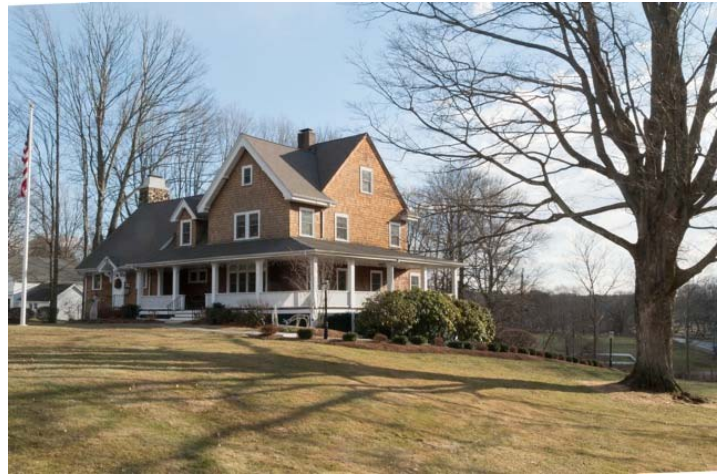
Main Street: 28 (Southborough Community House). View SE.
