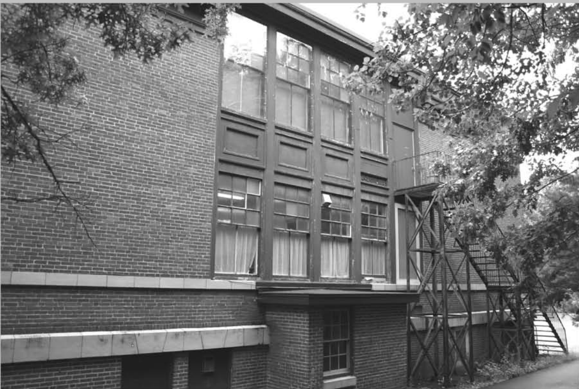
4. South Union School, rear (north) elevation. View SW.
