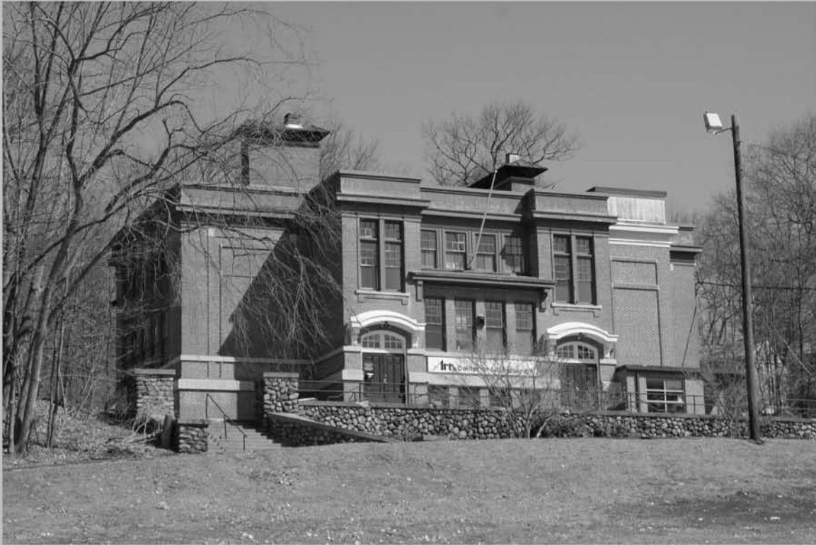
7. South Union School, façade (south elevation) and monumental stair. View NE.
