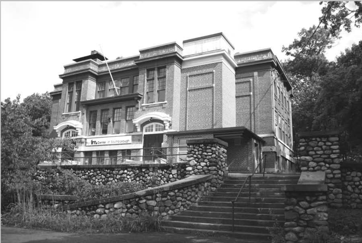
1. South Union School, façade (south elevation) and monumental stair. View NW.
