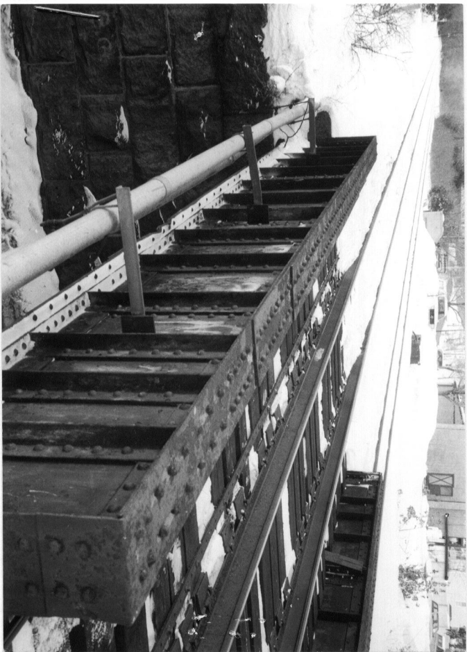
Rt. 85 Bridge under MBTA - south side plate girder.
