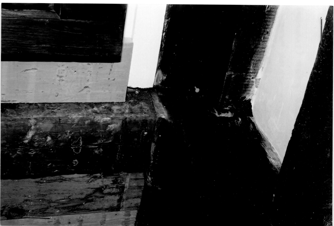
main house kitchen chimney girt and post (interior) note step of girt which runs from front to back of house
